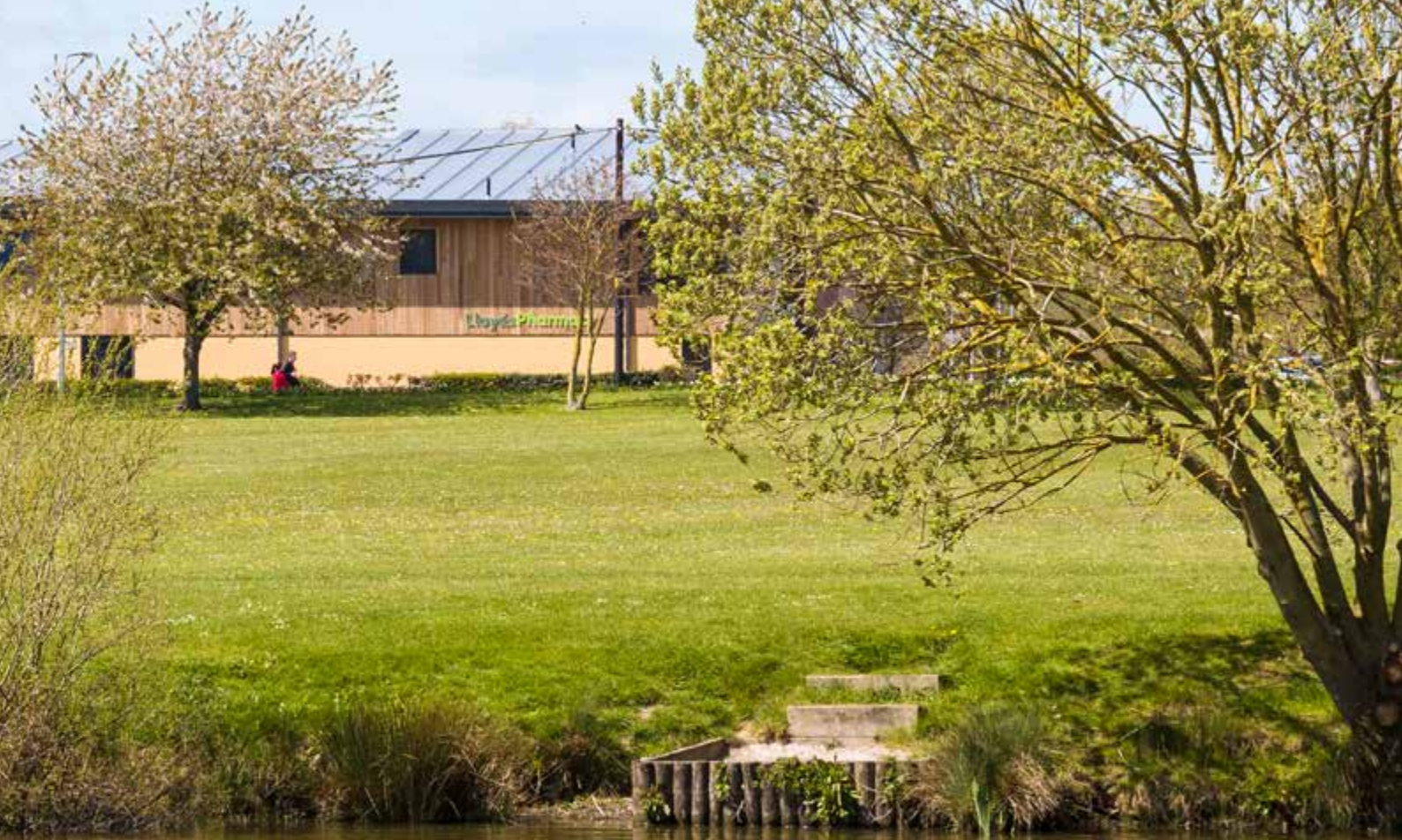
Buckley Medical Centre, Wales
